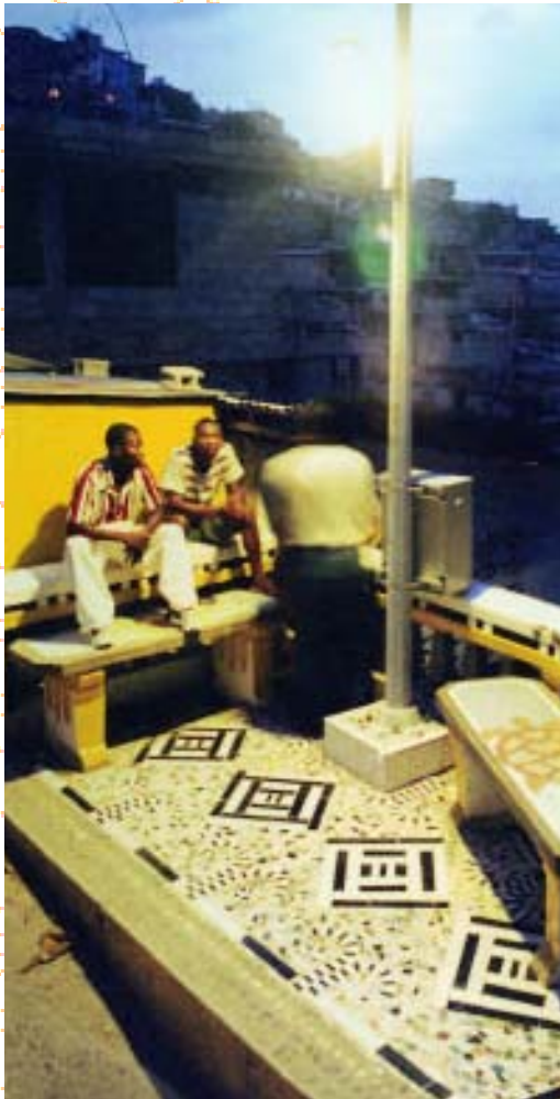
Meeting-place built and decorated by the residents of Jalousie in Port-au-Prince (Haiti). Alone of its kind in the neighbourhood, this public space is one of the fruits of the MOST Programme's "Cities" project. © G. Domenach-Chich, UNESCO
