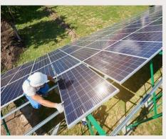
**Solar panel** is an assembly of photovoltaic cells mounted in a framework to produce electrical energy.
