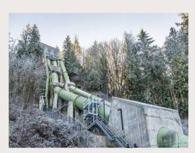
The forced pipe helps the water to reach the turbine at a higher speed.
