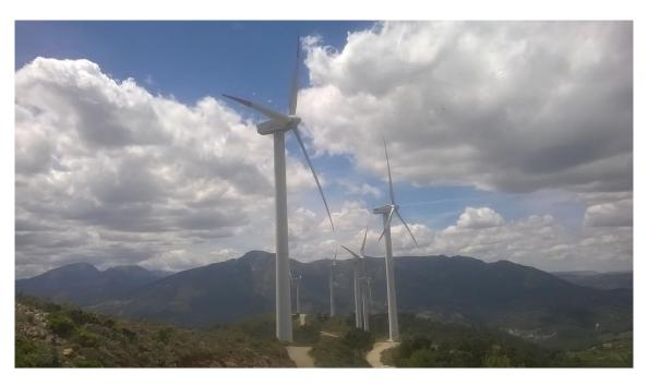
The wind park has a maximum power output of 15,300 kWh (kilowatt-hour) at any given moment, and operates an average of between 2,000 and 3,000 hours per year. If it produces 15,300 kWh 8,760 hours per year, that would be 100%, and 3.000 hours per year would be 34.25%. It could supply a town of 5,000 complete homes of three or four members.
