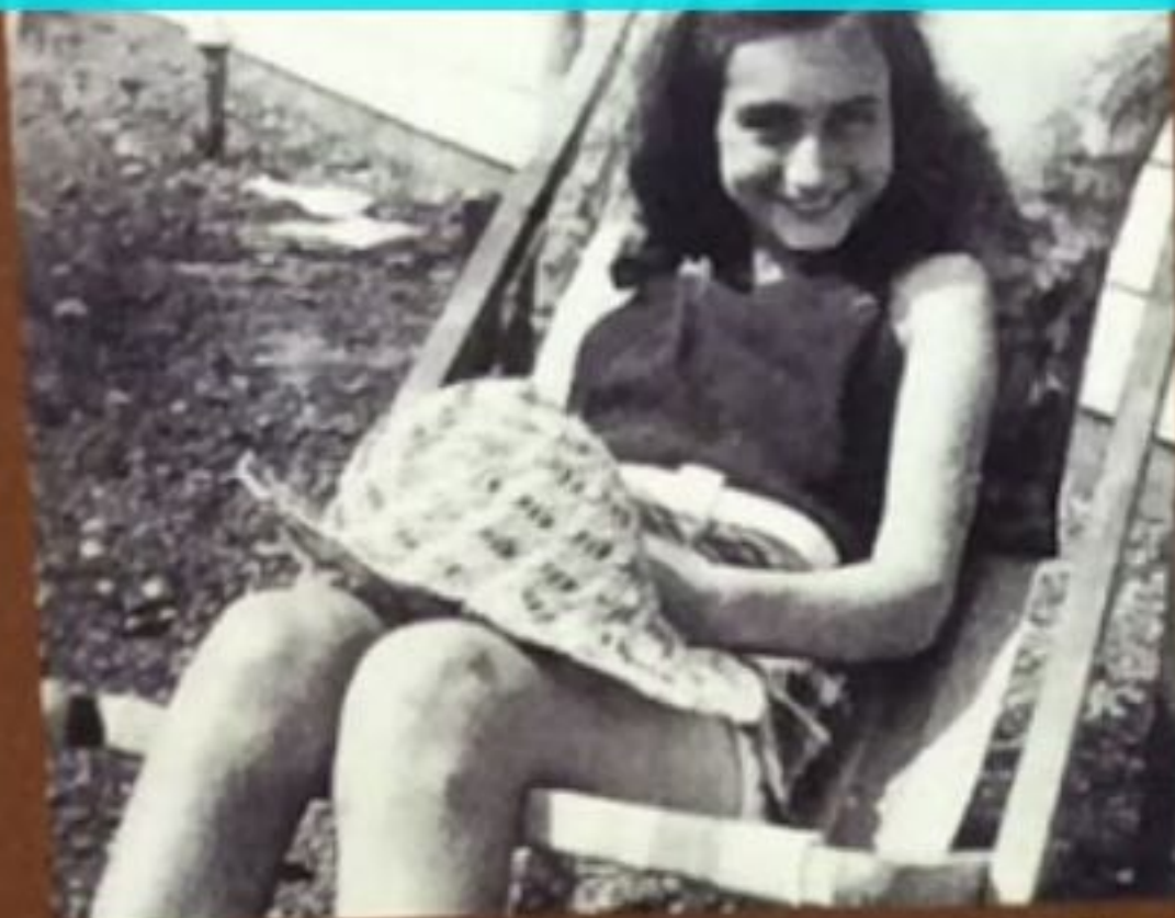
Anne on the flat roof of her house on the Merwedeplein square.
