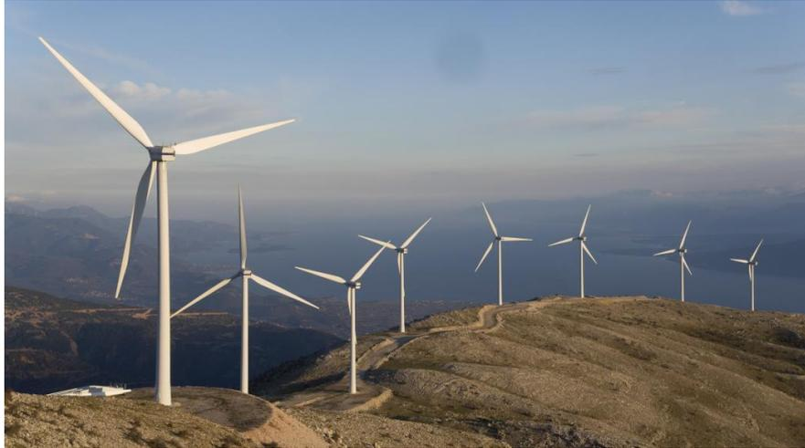
**Wind power generation** is quite unpredictable. For this reason, it is necessary to examine the wind potential from the wind potential mapping maps or even better to make wind speed measurements for at least a period of 6 months. The main parameter that determines the efficiency of the system is the average wind speed and its distribution on which depends the electricity that will be produced by the system per installed kW on an annual basis.
