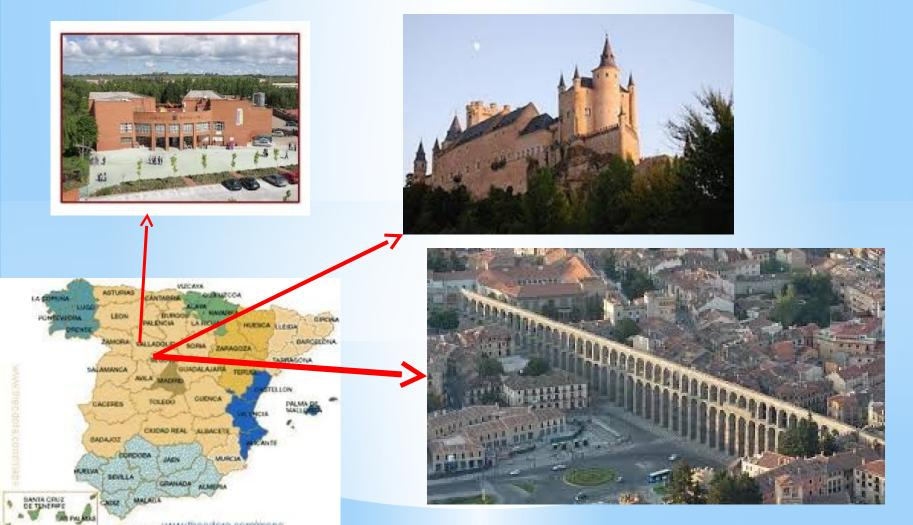
The first section of the aqueduct contains 36 semi-circular arches, rebuilt in the 15th century to restore a portion destroyed by the Moors in 1072. The line of arches is organized in two levels, decorated simply, in which predominantly simple molds hold the frame and provide support to the structure without any glue! On the upper level, the arches have width of 5.1 meters. The top of the structure contains the channel through which water travels, through a U-shaped hollow.
