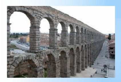
The aqueduct is built of unmortared, brick-like granite blocks. During the Roman era, each of the three tallest arches displayed a sign in bronze letters, indicating the name of its builder along with the date of construction.
