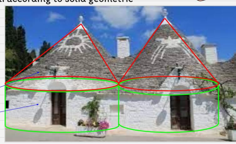
The roof is covered with chiancarelle thin slabs of limestone).
