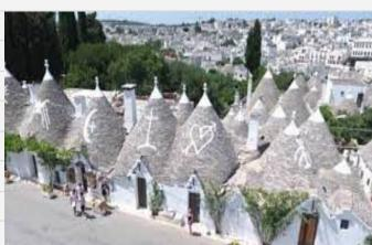
The typical trulli of Alberobello are mainly with a quadrangular plan and a plastered base. It's a primitive architectural typology that exploited the specific abundance of some limestone formations suitable as building material. Their origin is very ancient, the oldest trullo of which we know dates back to 1559.
