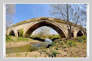
It is a stone arch bridge built by Mimar Sinan by Sokullu Mehmet Pasha in the second half of the 16th century. The bridge is 123 meters long and the span of the central arch in the form of a parabola is 20 meters.
