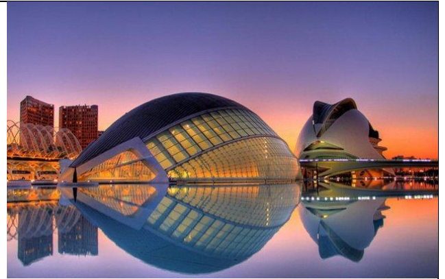
7. City of Arts and Sciences (València). Designed by Santiago Calatrava. Situated in the former riverbed of the river Turia.
