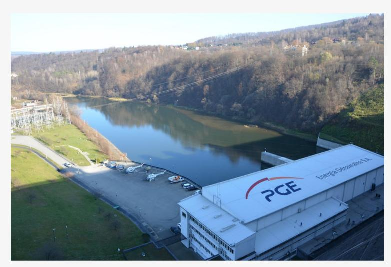
The Solina Dam (Polish: Zapora Solińska) is the largest dam in Poland. The dam is 664 m long, 8.8 m wide and 81.8 m high. Its construction created the largest artificial lake in Poland - Lake Solina. It has four turbines which are currently generating 200 MW of electricity.
