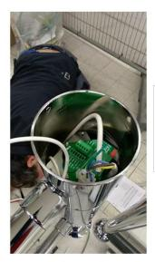
In this image, together with my employer we were mounting an electrical wiring of a sensoroperated electric gate
