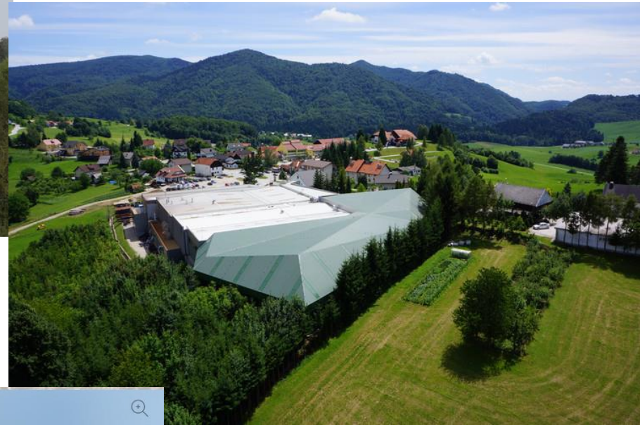
The Factory Tajfun – factory of forestry equipment
