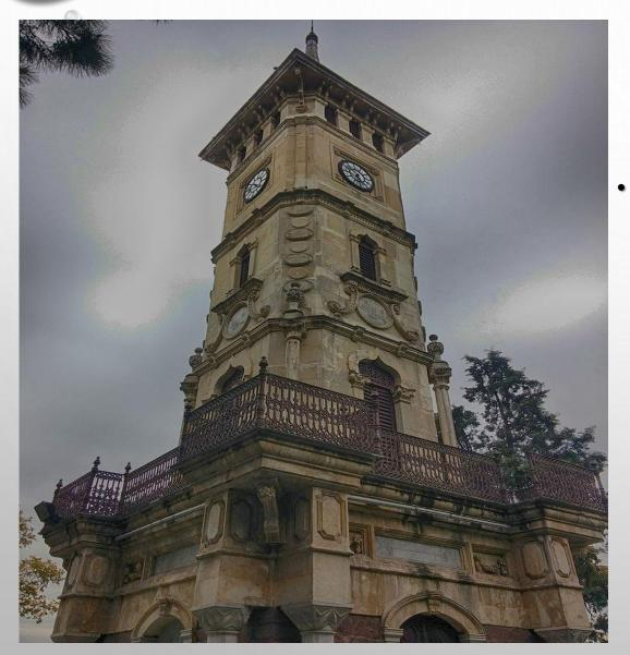
THE SIDES OF THE TOWER ARE IN THE FORM OF A SQUARE PRISM WITH BEVELED EDGES, ITS BODY RISES ON A 3.65 X 3.65 SQUARE PRISM. THE HEIGHT OF THE TOWER IS 16.4 METERS. IT IS DIVIDED INTO FOUR FLOORS, EACH WITH DIFFERENT ARCHITECTURAL PRACTISES AND DECORATIONS. THERE ARE TWO COLUMNS ON EACH CORNER OF THE PEDESTAL PART. THERE IS A PUBLIC FOUNTAIN ON THREE SIDES AND AN ENTRANCE DOOR ON ONE SIDE. IN THE UPPER PART OF THE COLUMNS WITH RHOMBIC SLICED CAPITALS, THERE ARE EIGHT-SEGMENTED, NESTED PANELS.
