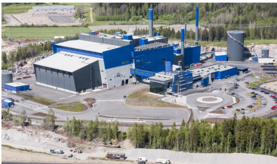
The newest waste incinerator in Vantaa, Finland.
