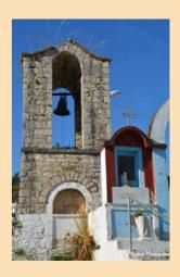
The building has two main building phases. The first phase dating back to 1847 belongs to the eastern part of the pedestal with the pillar. It is obvious that the stone wall of the cemetery was also built currently with the pillar. In the second phase, dating back to 1866, the pedestal took its final form and the present bell tower was built.
