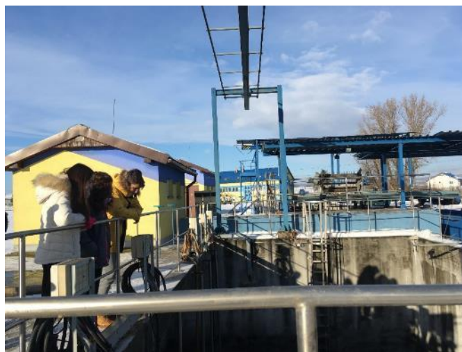
Visit to the water treatment plant in Humenné, Slovakia
