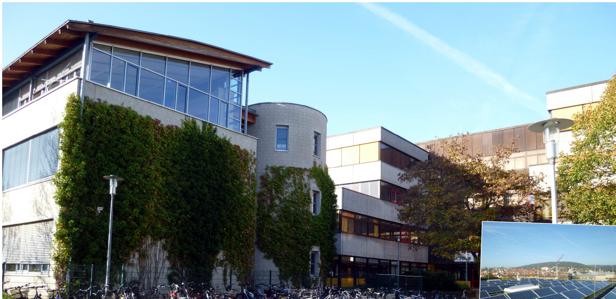
Germany: Main-Taunus-Schule in Hofheim, buildings and solar panels
