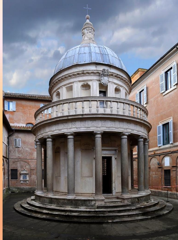
THE CLOISTER OF BRAMANTE
