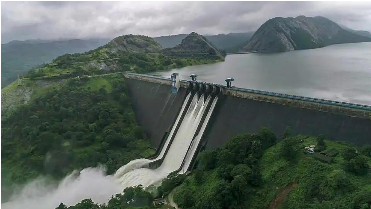
The water dam of Idukki in Kerala, in india reach in 2018, 90% of its capacity.
