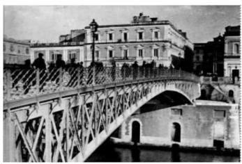
The structure was revised between 1957 and 1958: the turbines were replaced by an electrical system according to a project of the Società Nazionale Officine di Savigliano and the bridge was made entirely of metal.
