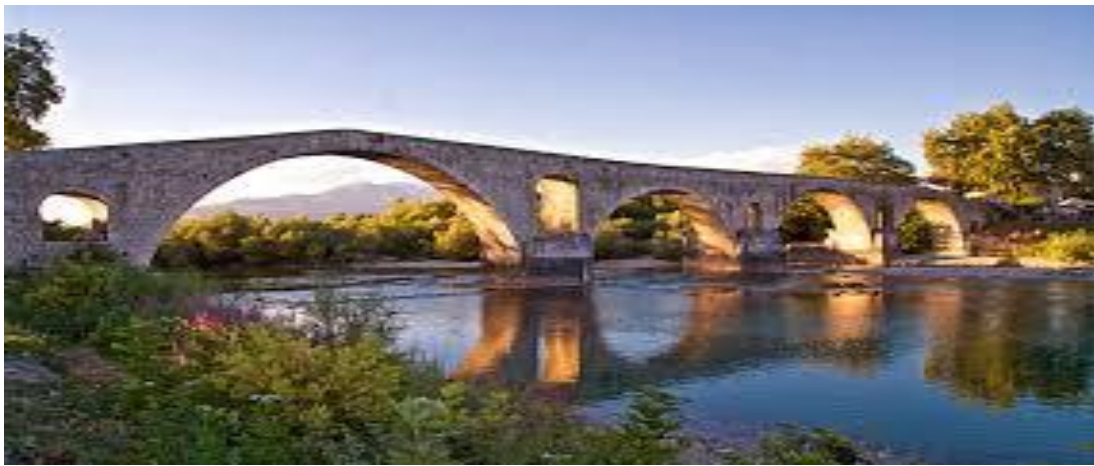
THE BRIDGE OF ARTA
