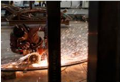
Steel Structures Factory, Portugal
