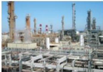
Galp Energia Refinery, Portugal
