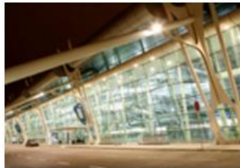
Francisco Sá-Carneiro Airport, Portugal
